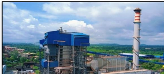
High Pressure –Cogen PP
